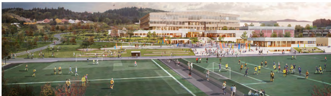
Starting from the beginning of the 2018 school year, students at Heimdal Upper Secondary School will be attending a school built for the low emission society (Illustration: Skanska/Rambøll).
